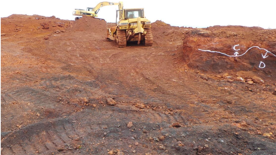
Nabeba trial mining area with stockpiling of iron ore material
