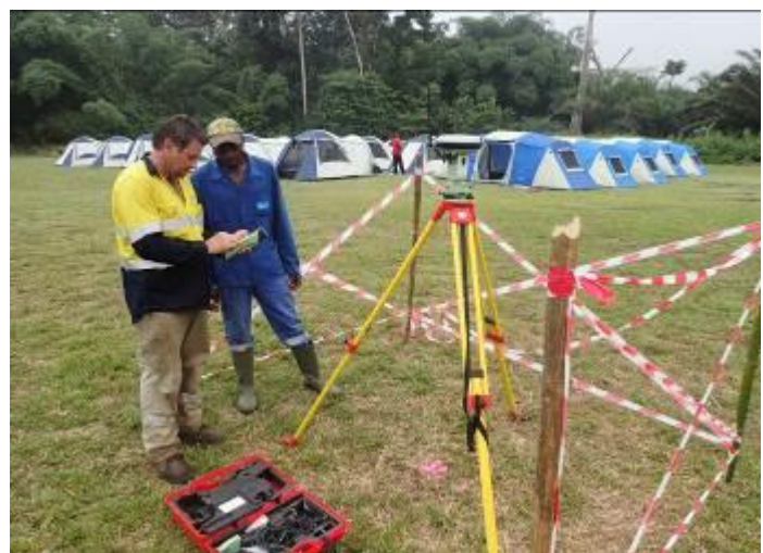
Surveying Activities and Field Camp on the Railway DUP
